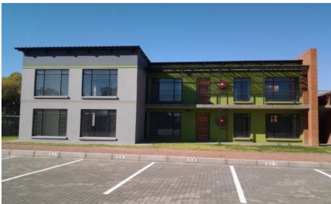
ZAMDELA CRU UNITS
