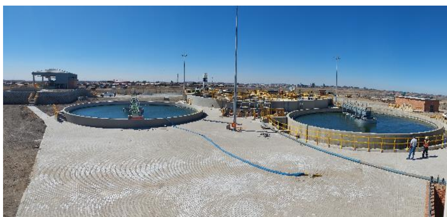
Upgrade of Refenggotso (Deneysville) WWTW Construction completed and the process of commissioning has been done
