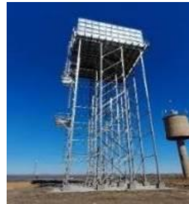
Upgrading of Orangeville WTW and Construction of Pressure Tower
