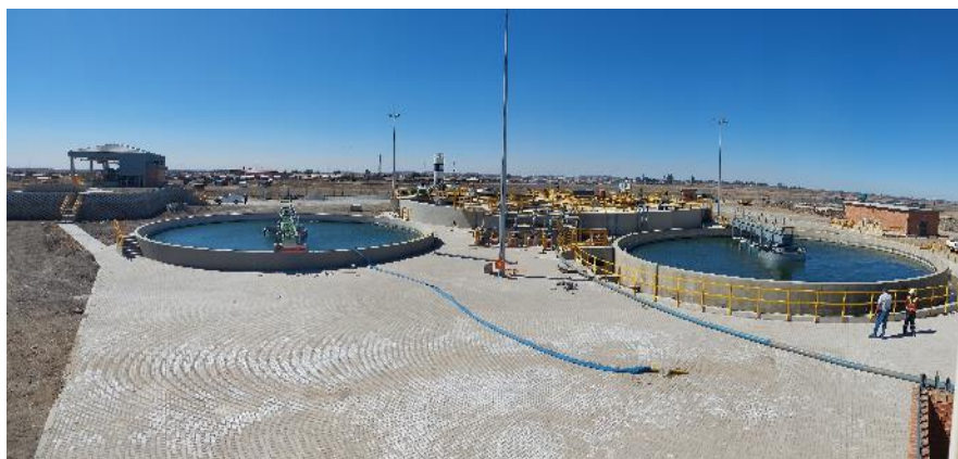
Upgrade of Refengkgotso (Deneysville) WWTW
