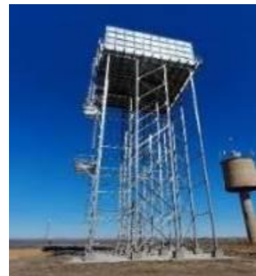
Upgrading of Oranjeville WTW and Construction of Pressure Tower
