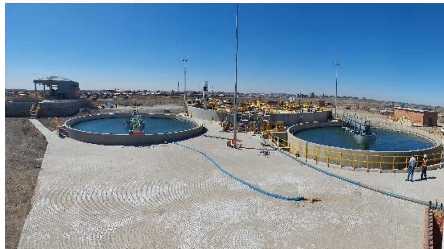
RBIG: Metsimaholo LM - Bulk Sewer Upgrade of Refengkgotso (Deneysville) WWTW
